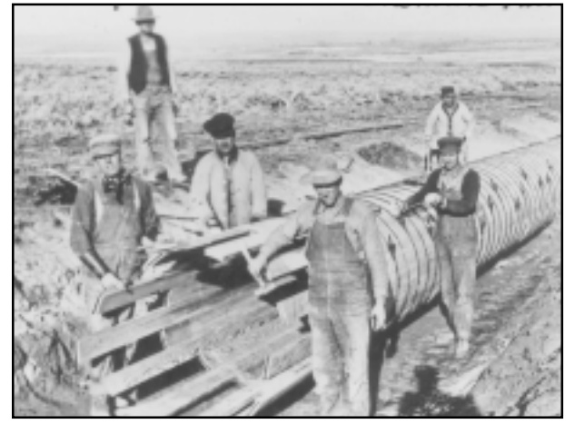
Building wood pipeline, March, 1912. Part of the Milner project. Idaho State Historical Society.
